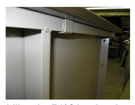
pool wall panel. The 90° angled bracket hooks under the outside of the panel top as shown in this photo.
