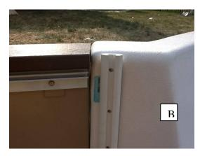
First locate the stair placement at the site. Insert the filler panel shown in photo "A". Align the appropriate panels to either side of the stair and clamp them to the stair flange. When using the "synthetic wood" top seat or the "PVC coping", the coping must be flush with the top of the stair as shown in photo B.
