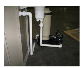
dealer for the proper sizing and filter media to meet your needs. When installing the plumbing lines, make sure that the skimmer is connected to the front (suction) of the pump and the return fitting is connected to the discharge side of the filter. Shut off valves are recommended for
