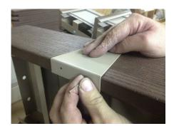
Locate the top cap joint covers and position them over each miter joint. Each cap hooks in the front first and secured to the top seat with color coated nails as shown.
