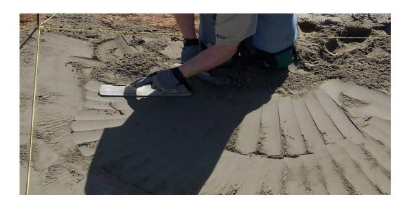
Spread the bottom material around the floor of the pool and compact it to just <u>cover</u> the string lines as you go. Use the edge of a flat board (about 36" long) to scrape the excess bottom material to expose the string lines. Run a trowel across the surface to smooth it out. A rounded bottom trowel works best. Remember to pull your pins and fill in their divots as you progress. "The last one out has to cover their tracks."
