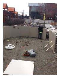
Secure the panels by using the 9/16" Galvanized nuts and bolts that were supplied with this package. Begin bolting the panels together using only the top two and the bottom bolt on each seam, until you have closed the circle. NOTE: Keep the panel connection on the outside of the layout stakes. We suggest that you hand tighten the panel bolts until the entire pool wall is erected.
