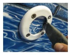
The return fitting face plate is installed in somewhat the manner as the skimmer. First find the round face plate and the pack of four faceplate screws supplied with the fitting.
