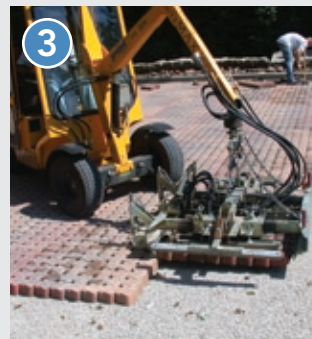
3 Install pavers at 5,000 sq. ft. (500 m 2 )/ machine/day
