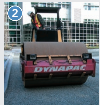
2 Spread aggregate base, sub-base and compact
