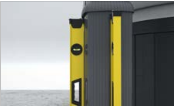
FIGURE 47: CHECK IF POSTS ARE STILL LEVEL
