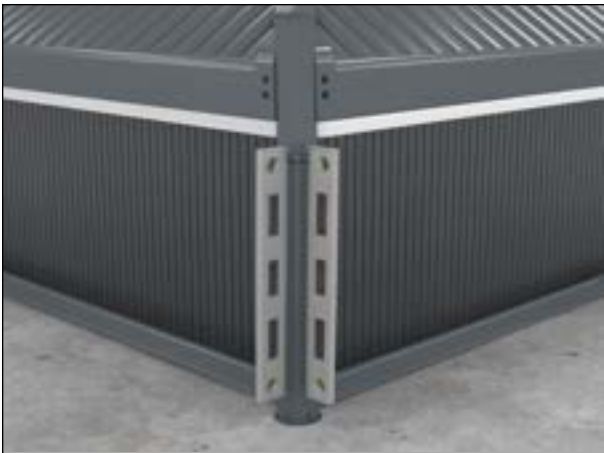
FIGURE 24: CHECK IF POSTS ARE LEVEL
